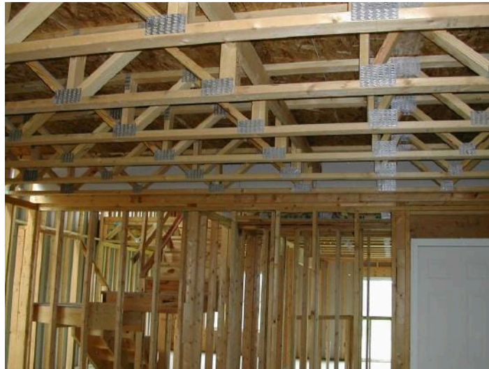
Figure 1.2.1: Floor trusses.
