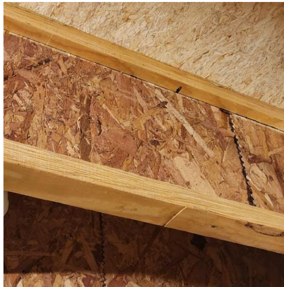
Figure 1.2.2: Lightweight engineered floor truss
