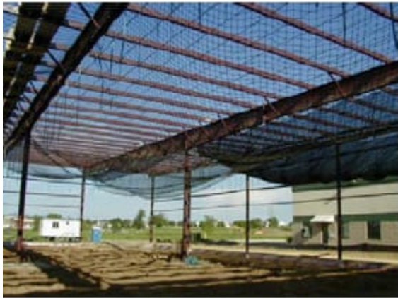
Safety nets used in construction sites.
