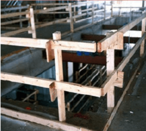
Properly installed guardrail system.
