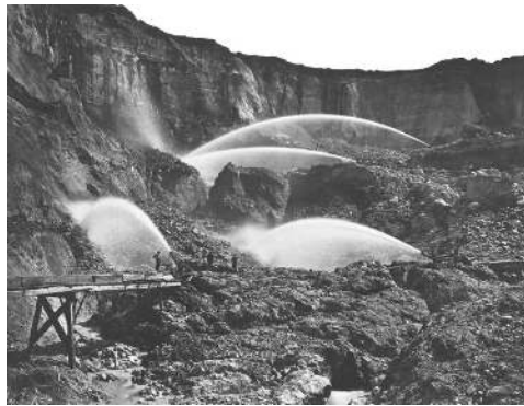
Figure 1.2.3.1: Hydraulic Gold Mining by Carlton Wakins is in the public domain - Hydraulic mining in the 1880s in Nevada City, California
