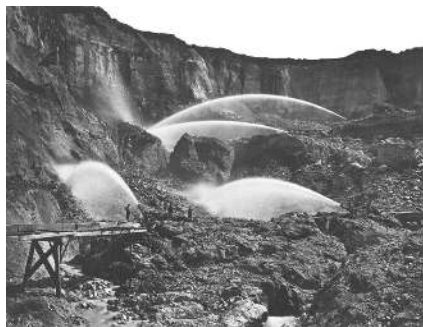
Figure 1.2.1: Hydraulic Gold Mining by Carlton Wakins is in the public domain - Hydraulic mining in the 1880s in Nevada City, California
