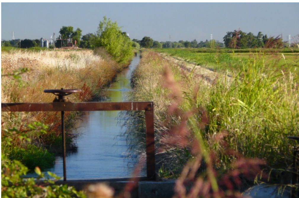
Figure Chapter 11.1: An Irrigation Ditch. (Copyright; Image by Bob White is licensed under CC BY-NC-ND 2.0 )
