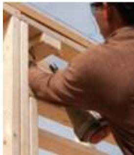
Figure 1.3.3: Nail penetration through the lumber is a special concern where the piece is held in place by hand. Nail gun by OSHA is licensed under Public Domain
