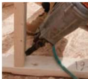
Figure 1.3.4: Toe-nailing by OSHA is licensed under Public Domain
