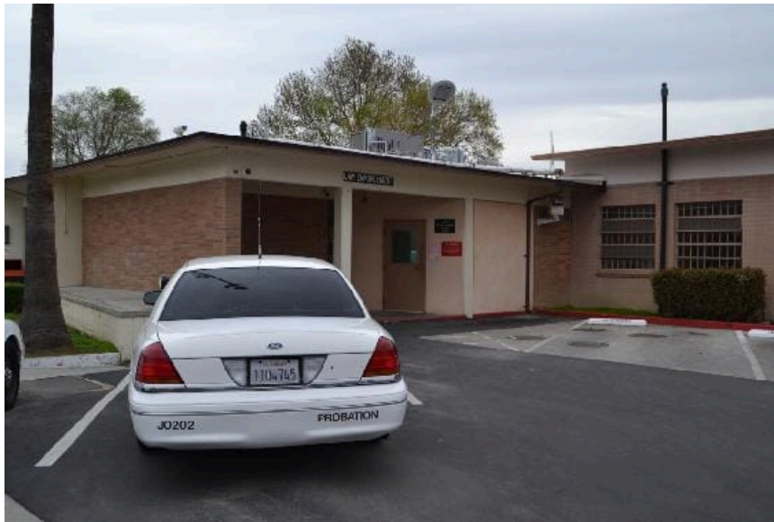
Figure 8.6 Law enforcement transport juveniles to detention facilities such as this to be booked. Security is a concern and officers must enter through a sally port. This is a secure area where the first door is locked before the second door can be opened into the facility. Booking photo by Tabitha Raber is used under a CC BY 4.0 license.
