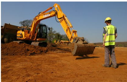
Figure 7.2.1: A back-hoe clearing topsoil from a site.
