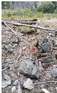
Figure 2 – This abandoned structure shows the effects of floralturbation (plants growing through the stairway) as well as faunalturbation. (The red arrow points to an animal burrow.) The rocks from the wall falling downhill also illustrate graviturbation. (Photo by the author.)
