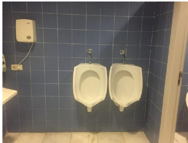
Figure 7.2.10: Inside a men's bathroom at a University in Madrid, Spain (CC By; Tom Grothe)
