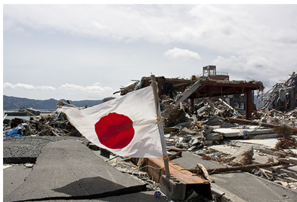
Figure 4.4.1: Devastation of March 11, 2011 earthquake in Honshu, Japan. (credit: Daniel Pierce).
