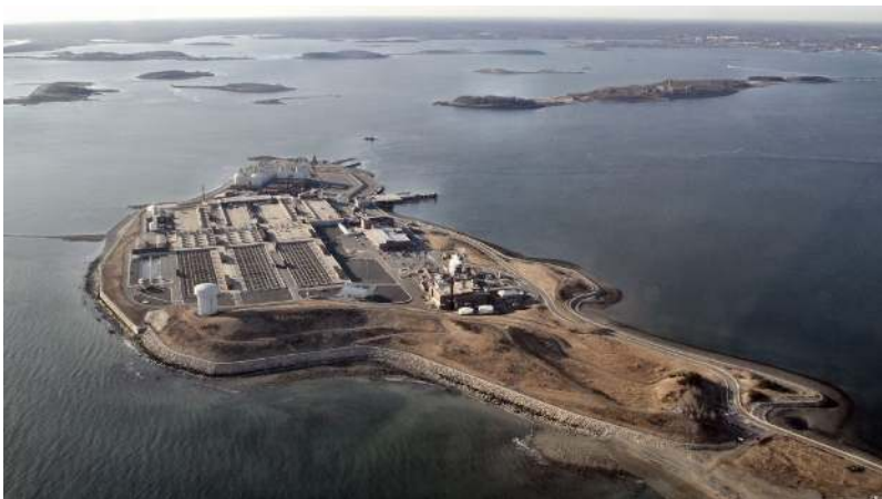
Figure 1.5: Deer Island in Boston Harbor is the current site of the city’s sewage treatment center. (CC BY-SA; Doc Searls).
