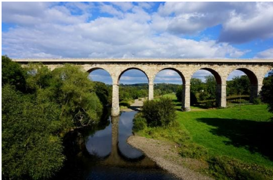
Figure 2.4.1 "bridge" barnyz is licensed under CC BY-NC-ND 2.0
