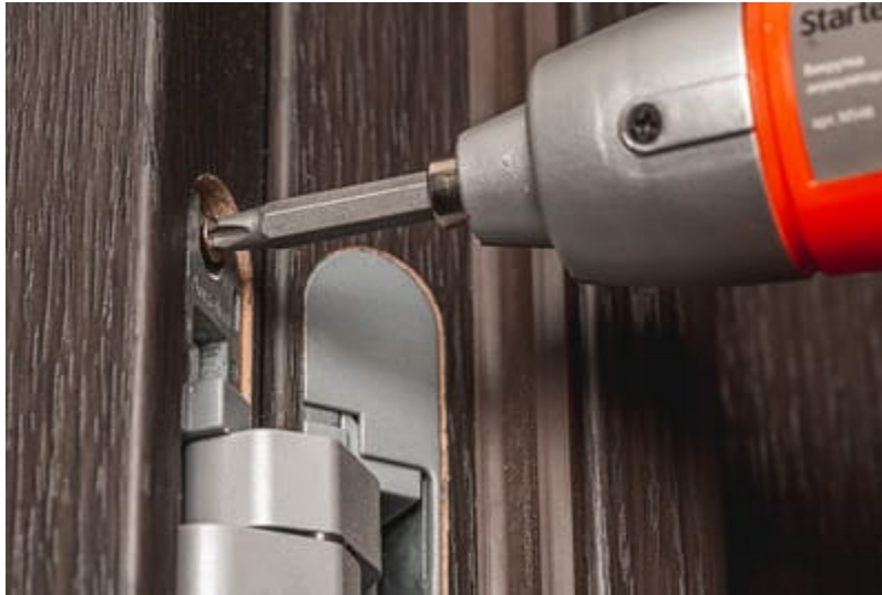
Figure 2.3.1: "Close-up, electric screwdriver secures the door hinge" by Marco Verch is licensed under CC BY 2.0.
