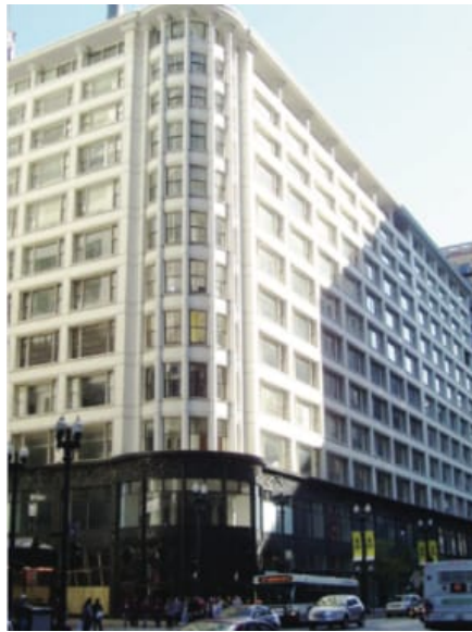
Figure 11.4.2: Carson, Pirie, Scott and Company Building, Chicago, IL. (CC BY-SA 4.0; by Beyond My Ken via Wikimedia Commons)
