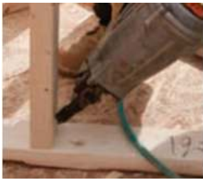
Toe-nailing by OSHA is licensed under Public Domain
