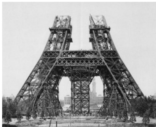
Eiffel Tower, Start of construction of second stage, May 1888. Image in the public domain
