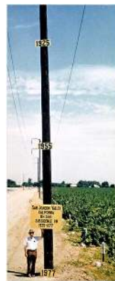
Figure 5.2: An Image of Maximum Subsidence in the San Joaquin Valley from 1925 to 1977.[2]
