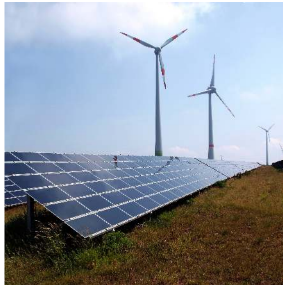
Figure 1.11.3: Photograph of Solar Panels and Wind Turbines.
