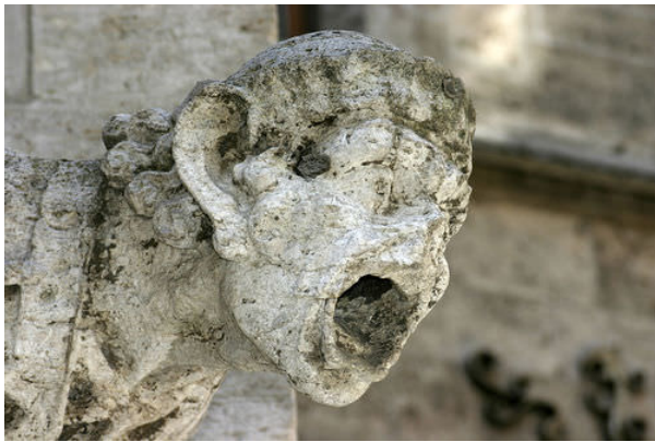
Figure 11.3.2: A gargoyle that has been damaged by acid rain.
