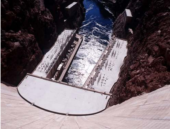
Figure 12.3.1: Hoover Power Plant View of Hoover Power Plant on the Colorado River as seen from above. Source: U.S. Department of the Interior
