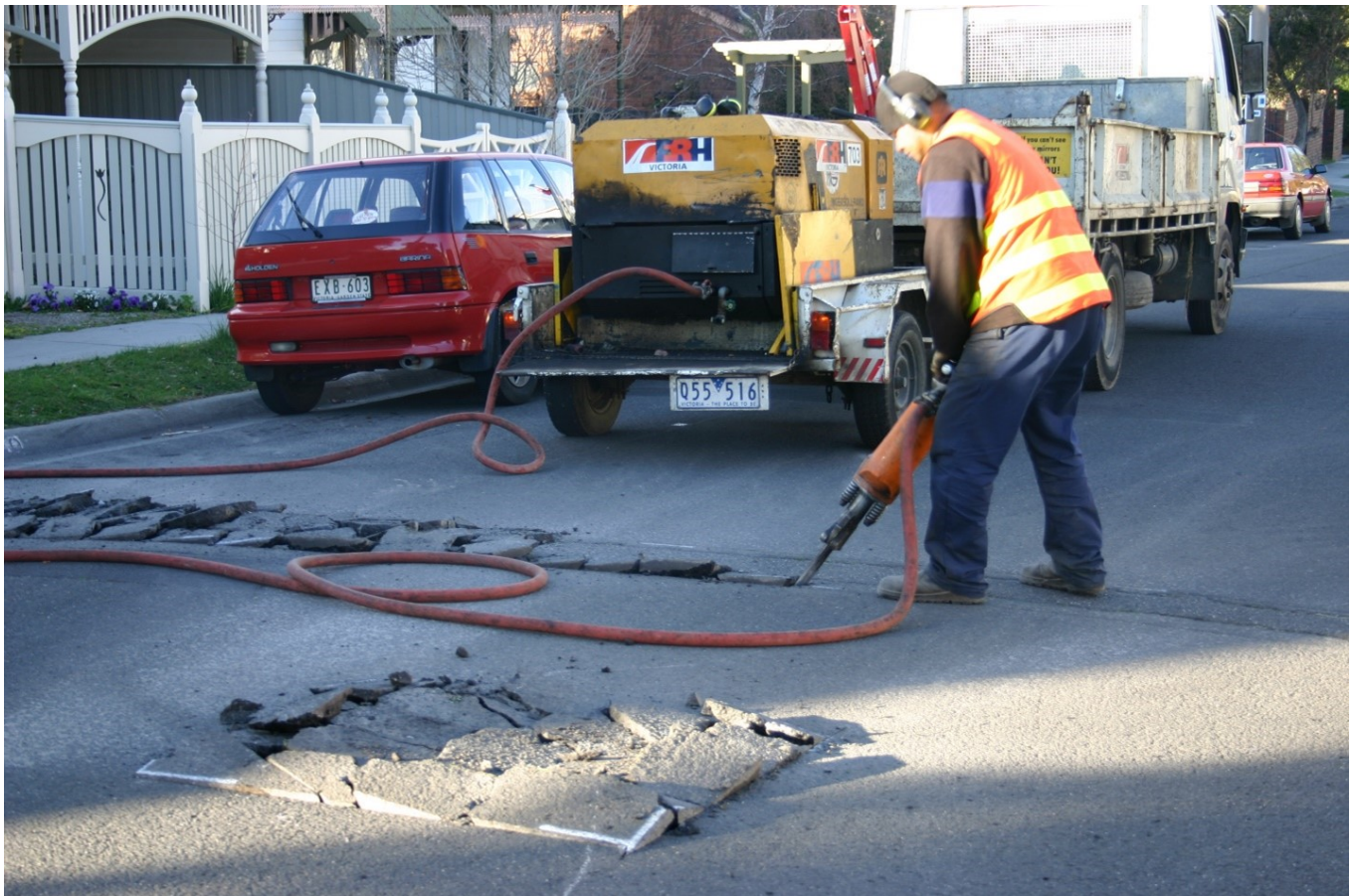
Figure 1.1.1: A man using a pneumatic jackhammer to break up asphalt. Original file by Josh Parris . Licensed under the Creative Commons Attribution 2.0 Generic license.
