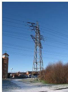
Figure 5.3.5: The power line tower also does not lie in a single plane and is therefore a space truss. Image by Anders Lagerås CC-BY-SA 2.5.
