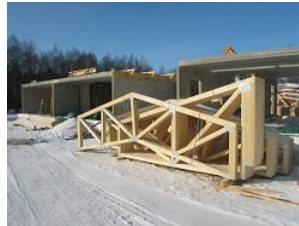
Figure 5.3.2: The members of these trusses all lie in a single plane. These roof trusses are an example of a plane truss. Image by Riisipuuro CC-BY-SA 3.0.
