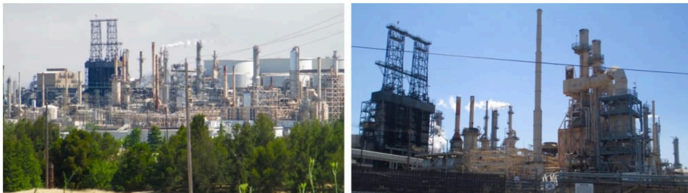
Figure 5.41: San Francisco Refinery in Rodeo, California.
