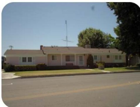
Figure 13.4.1: A home with a swamp cooler attached to the roof.
