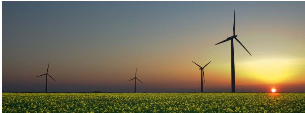
Figure 4.3.1: How many forms of energy can you identify in this photograph of a wind farm in Iowa? (credit: Jürgen from Sandesneben, Germany, Wikimedia Commons)
