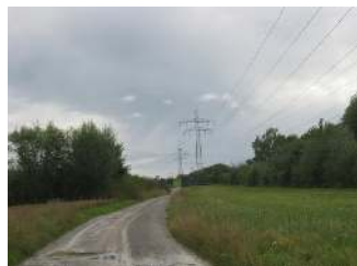
Figure 6.2.1.1.2: This high-voltage traction power line running to Eutingen Railway Substation in Germany radiates electromagnetic waves with very long wavelengths. (credit: Zonk43, Wikimedia Commons)
