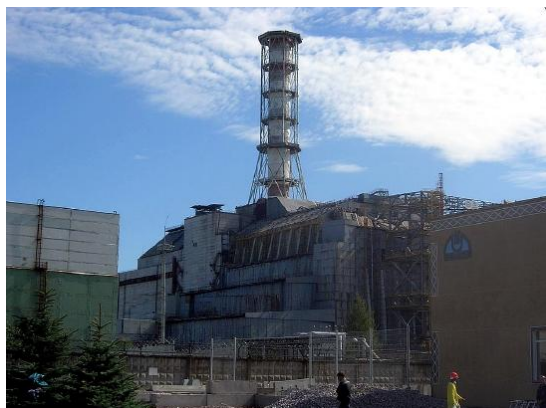
Figure 5.6.6.8: The Chernobyl reactor #4 building as of 2006, including the later-built sarcophagus and elements of the maximum-security perimeter. ( https://www.flickr.com/photos/83713082@N00/535916329/ ; Carl Montgomery )
