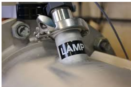
Figure 4.5.2: Ultraviolet lamp sanitizing water. Image courtesy of: https://www.nab.usace.army.mil/Media/News-Stories/Article/946068/army-water-treatment-plant-brings-a-unique-first/
