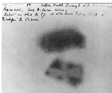
Figure 5.1.3: Image of Becquerel's photographic plate which has been fogged by exposure to radiation from a uranium salt. The shadow of a metal Maltese Cross placed between the plate and the uranium salt is clearly visible (Public Domain).
