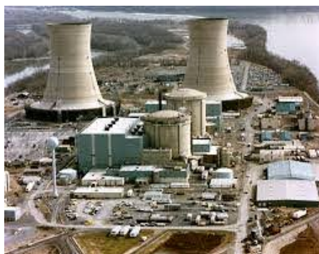
Figure 5.6.5.1: Color photograph of the Three Mile Island nuclear- generating station, which suffered a partial meltdown in 1979. The reactors are in the smaller domes with rounded tops (the large smokestacks are just cooling towers). (United States Department of Energy)
