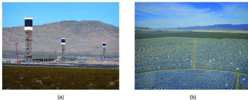
Figure 2.1.9: (a) The Ivanpah solar thermal plant uses 170,000 mirrors to concentrate sunlight on water-filled towers. (b) It covers 4000 acres of public land near the Mojave Desert and the California-Nevada border. (credit a: modification of work by Craig Dietrich; credit b: modification of work by "USFWS Pacific Southwest Region"/Flickr)
