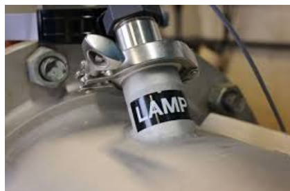
Figure 3.4.1.2 Ultraviolet lamp sanitizing water. Image courtesy of: https://www.nab.usace.army.mil/Media/News-Stories/Article/946068/army-water-treatment-plant-brings-a-unique-first/
