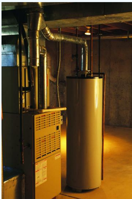
Figure 8.11.2 Tank water heater © Thinkstock. Most homes in the United States have a tank-type water heater like this one.
