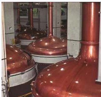
Figure 8.4.3: An oxide of carbon is removed from these fermentation tanks through the large copper pipes at the top. (credit: "Dual Freq"/Wikimedia Commons)
