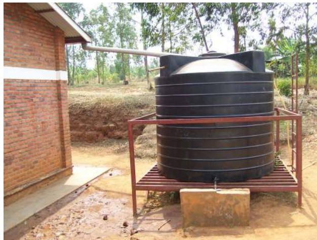
Figure 4.14: Rainwater harvesting storage tank example.
