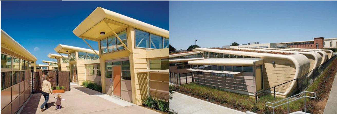
Figure 15.1.1: Project Frog Modules Linked to Make the Child Development Center, City College of San Francisco
