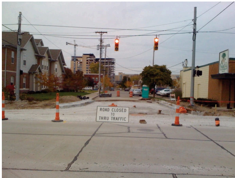
Figure 7.1.1: A Typical Construction Site
