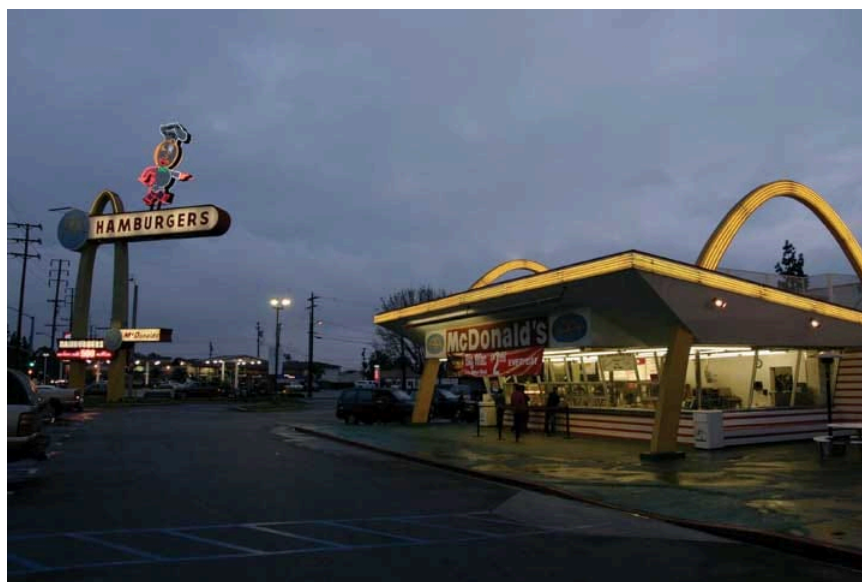
Figure 7.16: The oldest operating McDonald's is in California.
