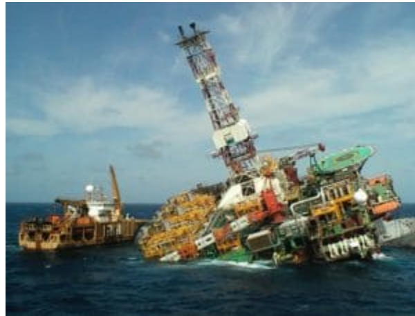
Figure 2.4.: The Petrobras P-36 oil platform sinking.
