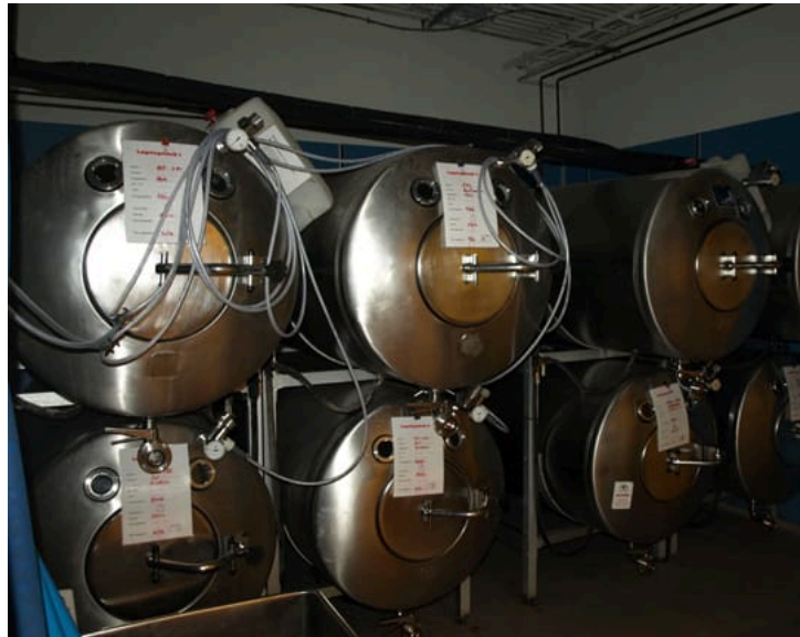
Figure 10.4.3: Fermentation of grape juice to make wine produces \text{CO}_2 as a byproduct. Fermentation tanks have valves so that pressure inside the tanks can be released.
