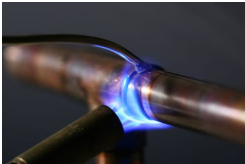
Figure 3.4.4: Propane torch being used to solder copper pipes for residential water mains. Source: Kevin L Neff / CC BY ( https://creativecommons.org/licenses/by/2.0 )
