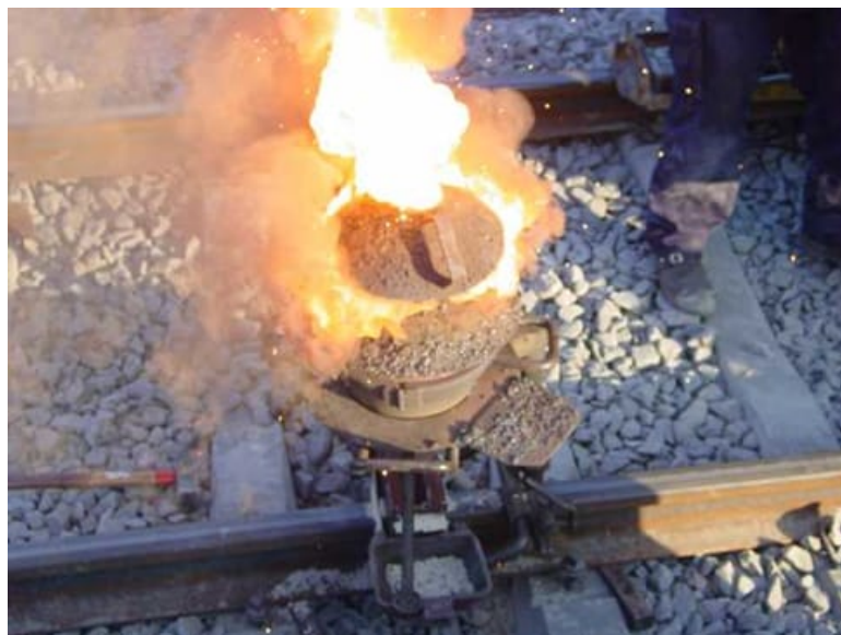
Figure 3.4.1: Thermite reaction proceeding. Shortly after this, the liquid iron flows into the mold around the rail gap. Source: http://en.Wikipedia.org/wiki/Image:V...ewelding-1.jpg , Public domaine.
