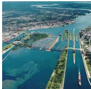
Aerial picture of the Soo Locks between Lake Superior and the lower Great Lakes in Sault Ste. Marie, Michigan, USA
